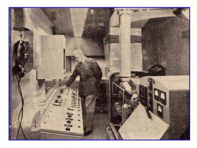
Two diesel AC generators are on the right side of car, can supply enough power to operate the train in any capacity.
