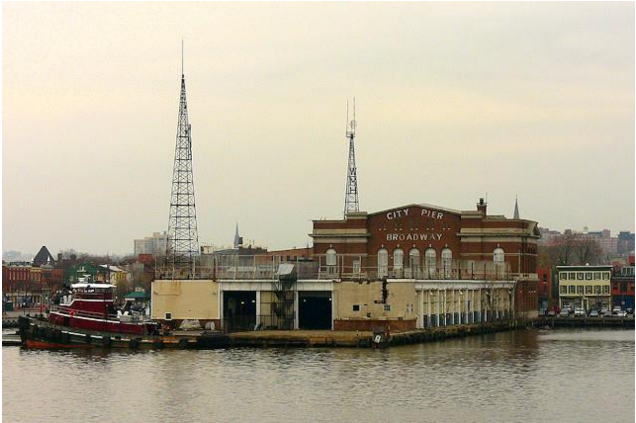
Figure 38: Coastal Station WMH Baltimore, Maryland
